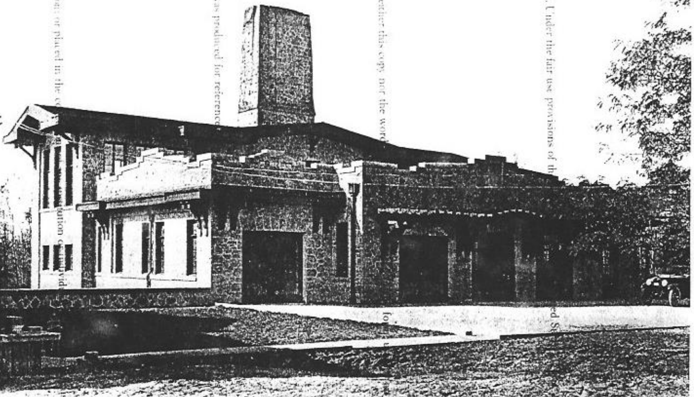
Garage, Power House and Laboratory. HOUSE, HENRY FORD, DEARBORN, MICH.
